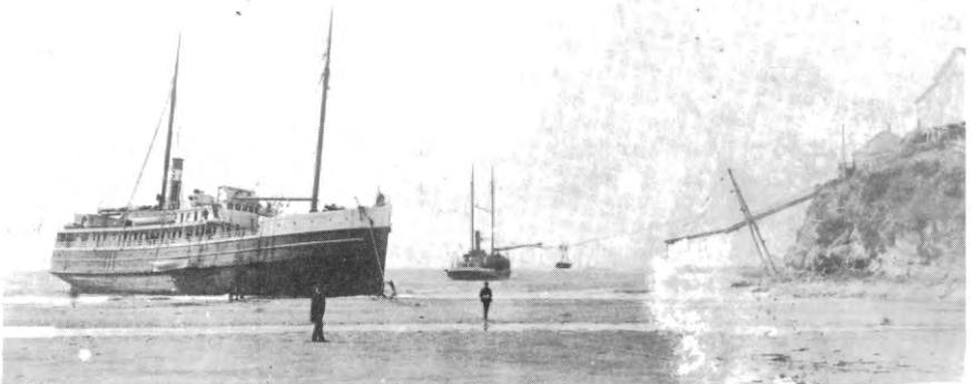
Steamer "Alliance" ashore at Caspar, April 5, 1903, with a steam schooner in background loading from Caspar Lumber Company wire chute. Note wooden chute closer to shore for loading to deck of vessel by a slide-system.
