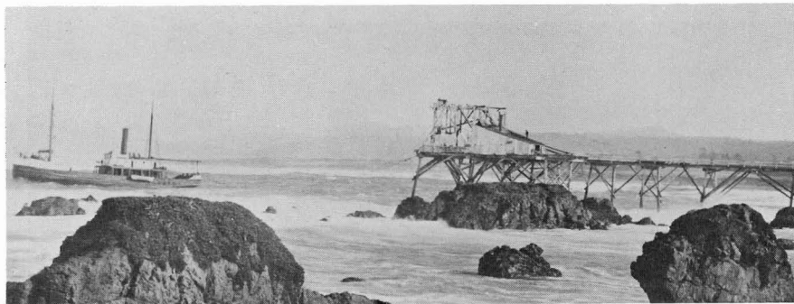
The Laguna Chute of the Little Valley Lumber Company with the steam schooner "Sequoia" loading.
